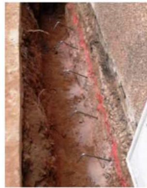
P4 – Dowel bars into existing foundations
