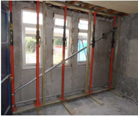
P7 – Ground floor propping (prior to erection of security screening)
