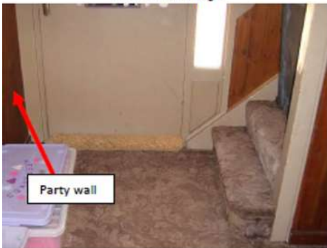
P5 – Staircase running parallel to the front wall (see also P9).
