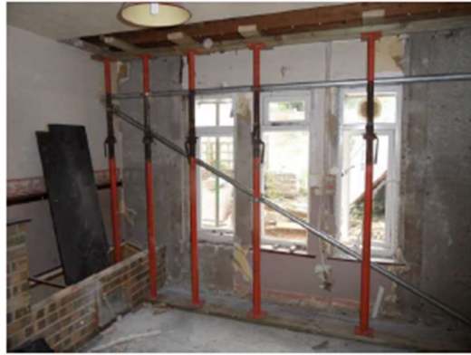
P8 – Ground floor propping (prior to erection of security screening)
