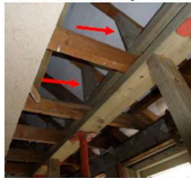
P6 – First floor propping with vertical support to roof rafter
