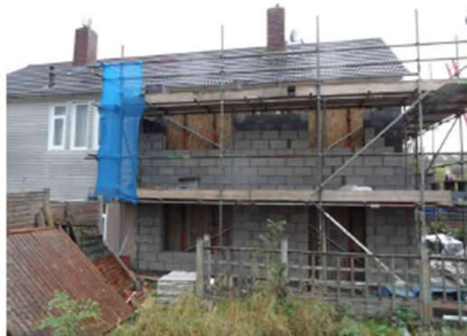
P12 – External Walls
