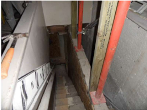
P9 – Propping on stairs (security screen at ground floor, first floor to be erected)
