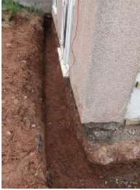
P1 – Excavation for foundation extension
