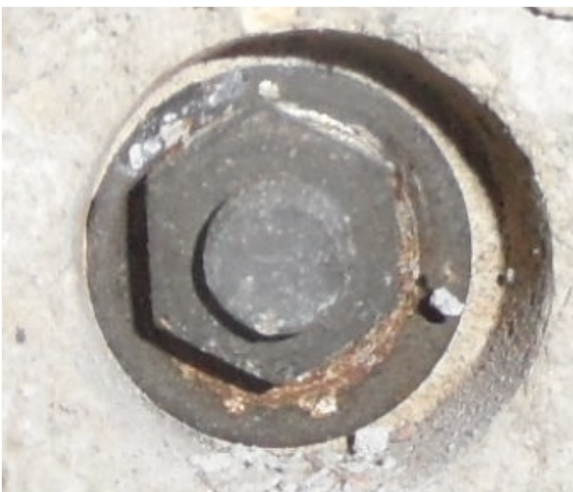
R17 – Panel fixing bolt
