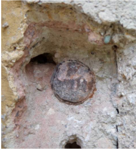
R13 – Bolt head at fixing between panel and column
