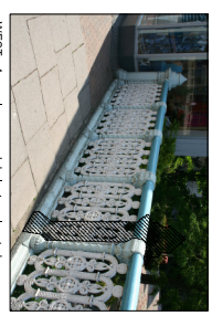
WEST - 4 panels removed, balustrade relocated
