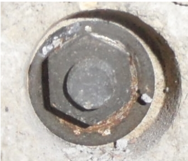
R17 – Panel fixing bolt
