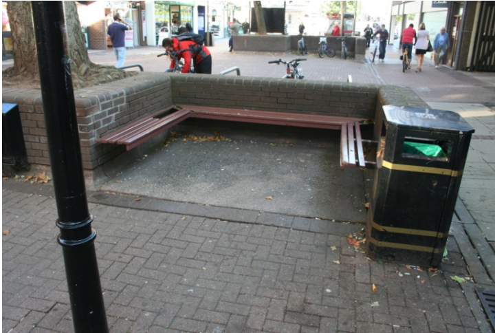
Dark brick planters, broken seats, litter and leaf catch
