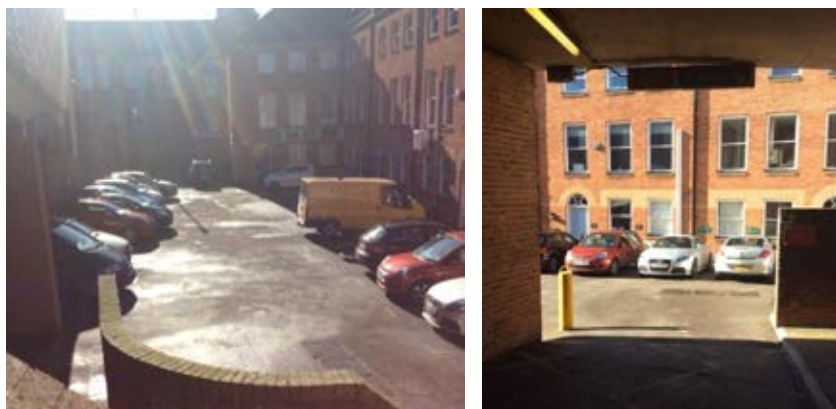
Figure 5, Private car park at rear of High Street MSCP
