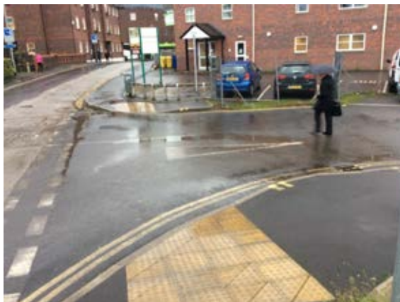
Figure 9, Castle Street Car Park entrance
