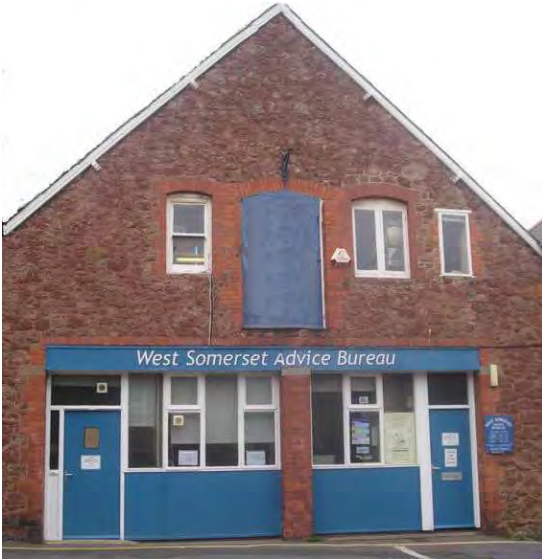
Picture of Building frontage before the building work had been done
