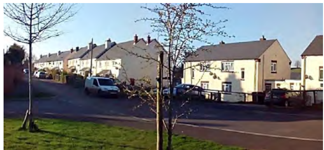
Slade Close looking West
