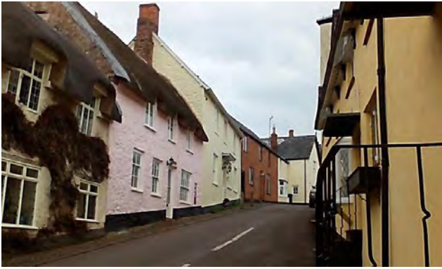
High St looking East Cobbled pavement on left; slate gully on right
