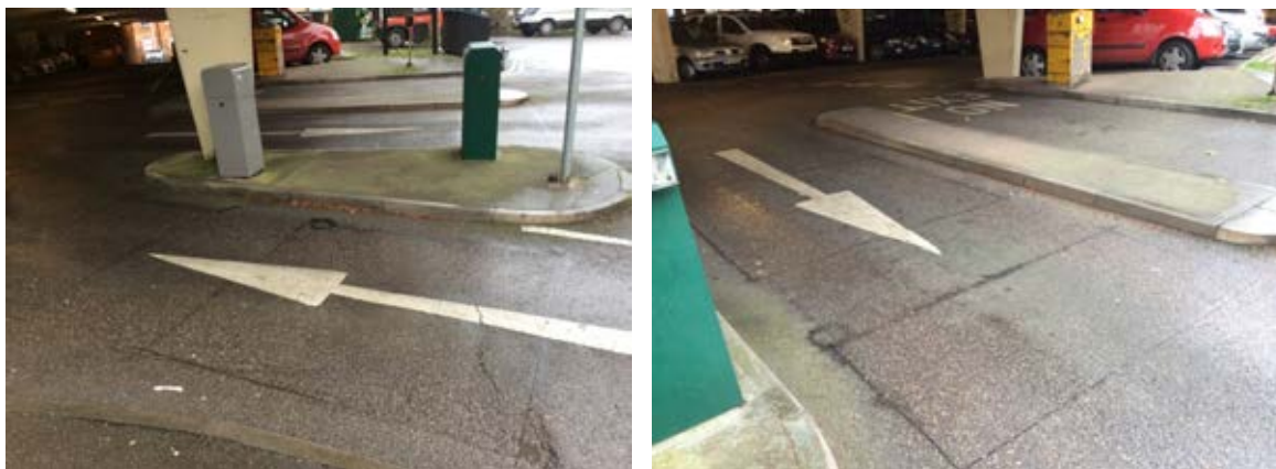
Figure 4, High Street car park entrance and exit lane views
