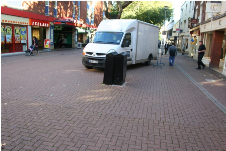
Isolated electrical boxes, loose, vulnerable & potentially dangerous
