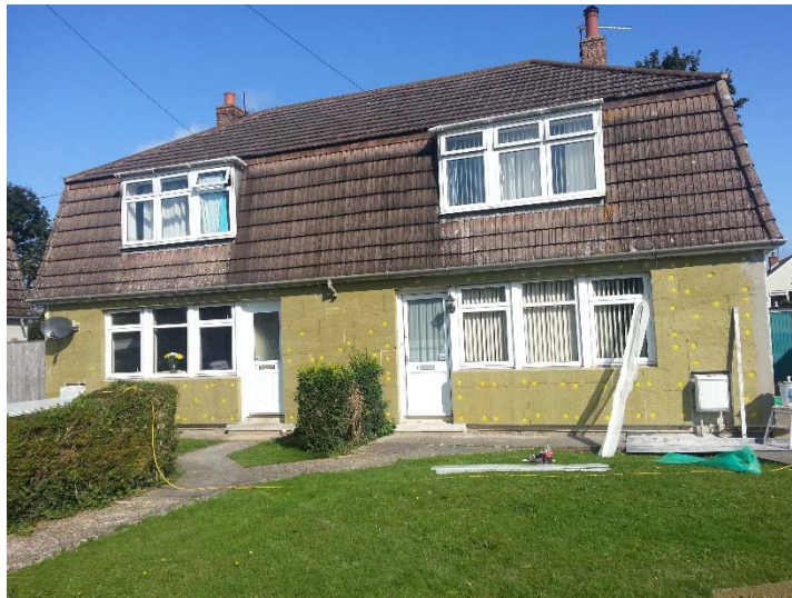
Insulation boards before render is applied
