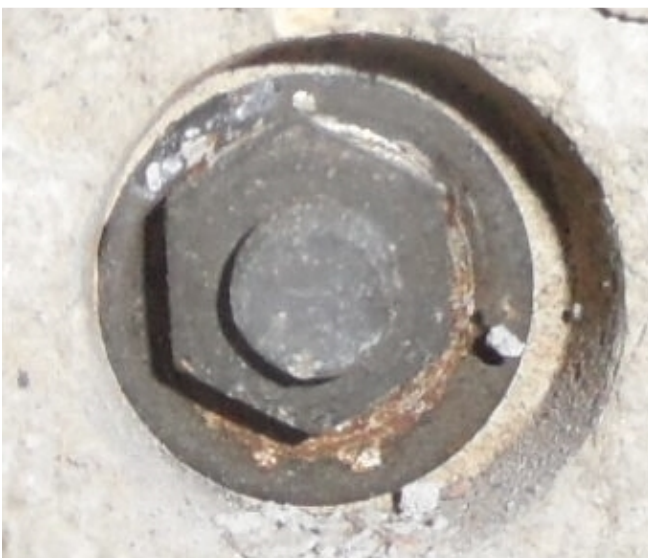
R17 – Panel fixing bolt
