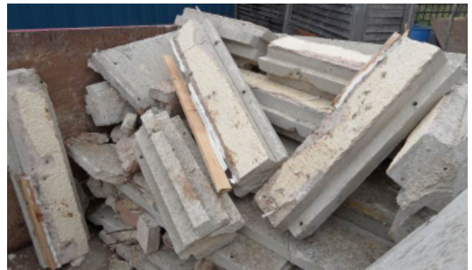
R18 – External wall PRC after dismantling for refurbishment works
